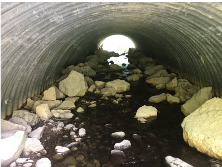
Looking through from inlet
